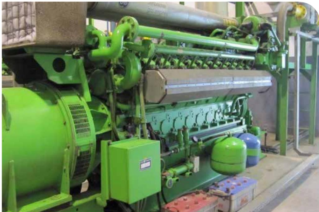
Gambar 4.26: Mesin gas Jenbacher 1MW di Bantar Gebang
